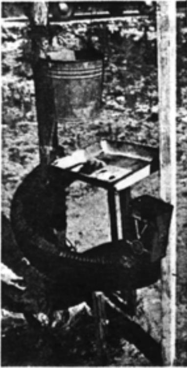
Some of the first testing for use of spiral process with ilmenite was done with simulated spiral made from old rubber tire before Trail Ridge mine construction began.
