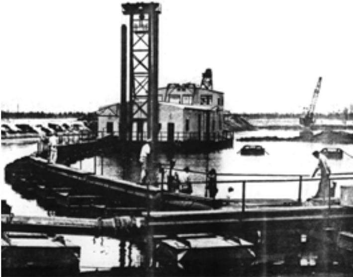
Dupont's original dredge makes picturesque scene as it eats its way through ilmenite ore body in "moving lake." This dredge was replaced early this year by new dredge with larger capacity.
